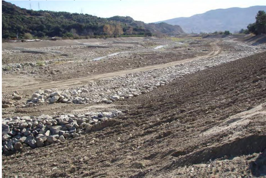
Figure 4-13: Emergency bank protection spur dikes.
