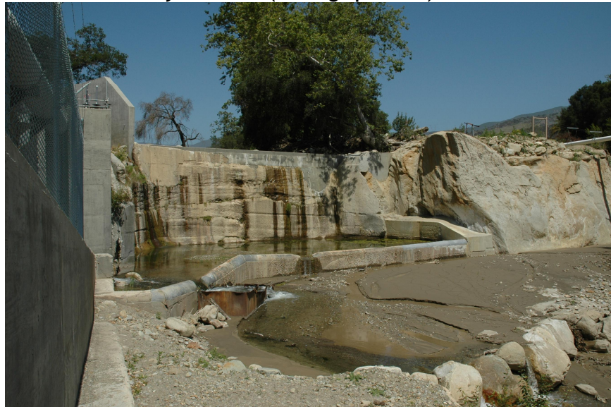
Figure 4-11: Below the Harvey Diversion (looking upstream).
