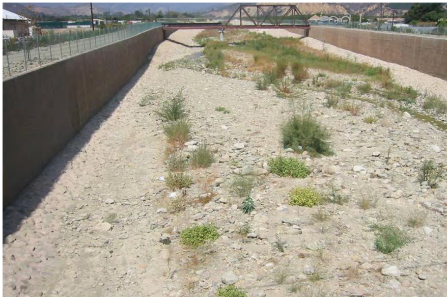
Figure 4-15: Looking downstream at the Southern Pacific Transportation Company (SPTC) truss bridge.
