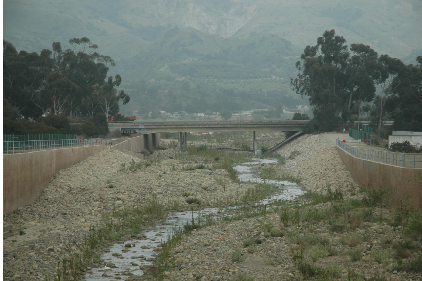
Figure 4-14: View of the existing USACE channelization (looking downstream at Hwy 126 crossing).
