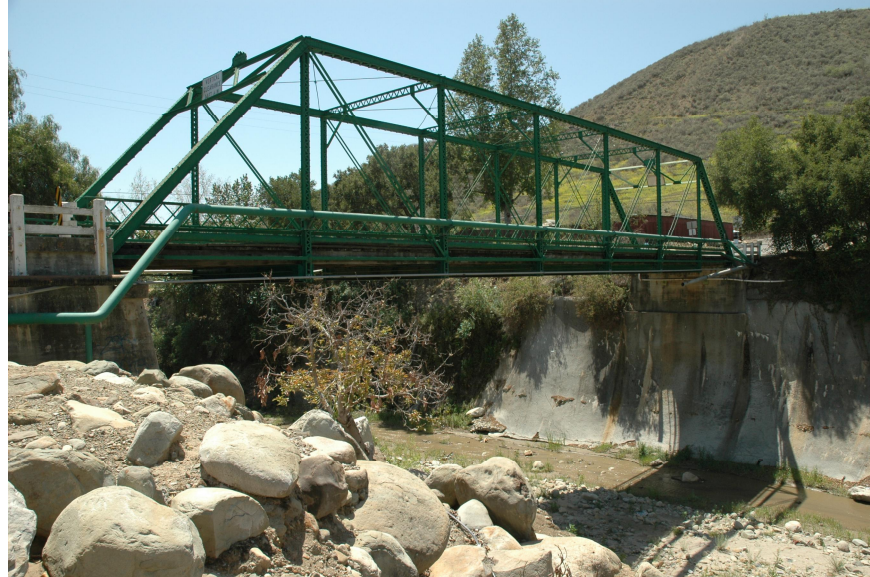
Figure 4-12: Bridge Road Bridge crossing of the confined stream reach.
