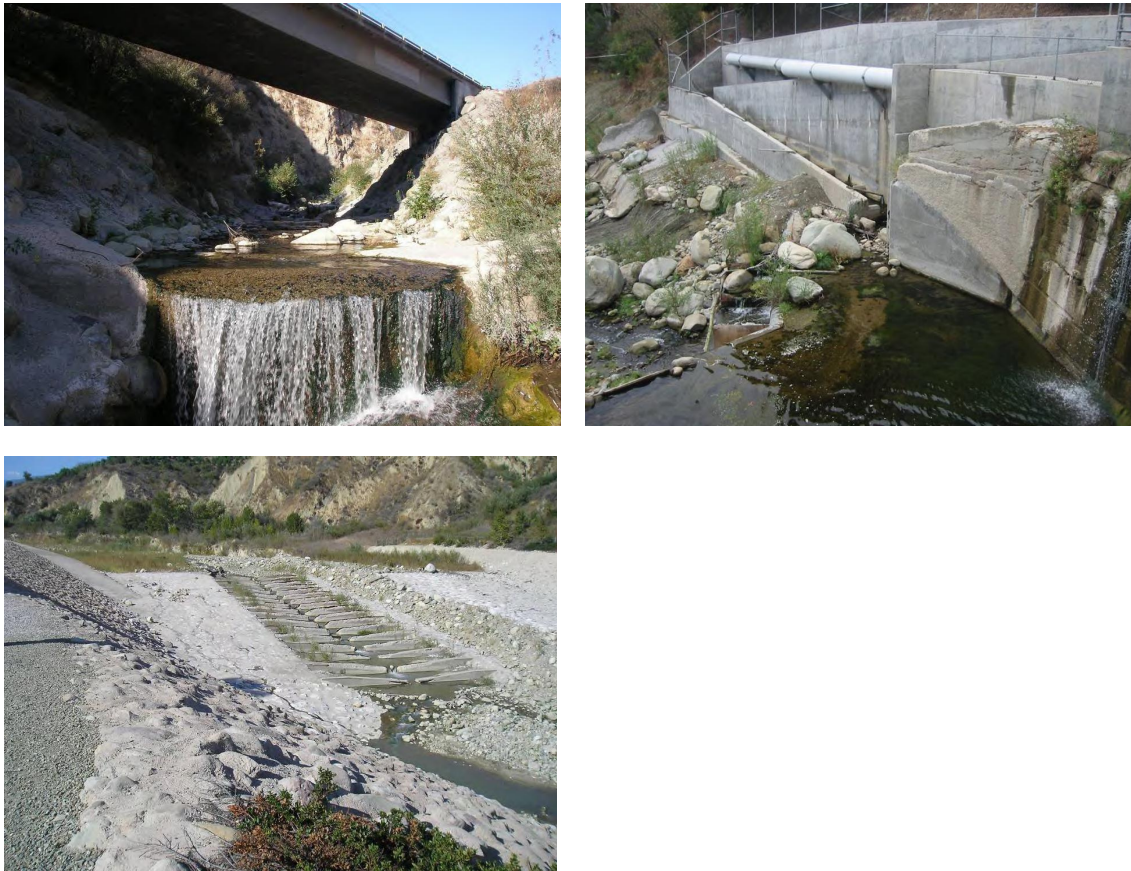
Figure 4-2: Photographs of damaged fish ladder facilities (from left to right, Hwy 150 Bridge, Harvey Diversion, USACE Fish ladder).
